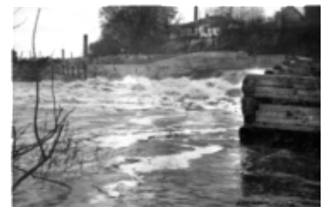
AFC 465-S13-I20 Floods on the Thames 4. -- ca. 1905-1912. -- 1 b&w photograph (tiff, jpg)
