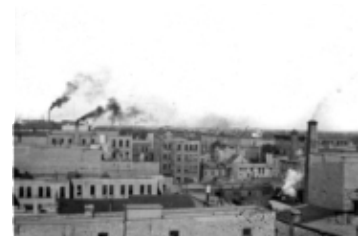
AFC 465-S4-I6 View 5th floor Smallman and Ingram [other Downtown buildings] 4. -- ca. 1905-1912. -- 1 b&w photograph (tiff, jpg)
