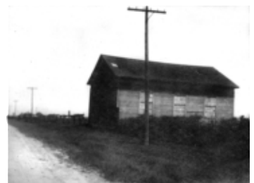
AFC 465-S7-I10 old Methodist church Gladstone. -- ca. 1905-1912. -- 1 b&w photograph (tiff, jpg)
