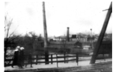
AFC 465-S13-I14 Flood time South Branch 1912 [Thames River]. -- 1912. -- 1 b&w photograph (tiff, jpg)
