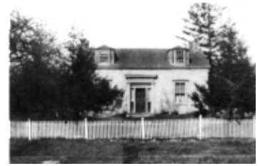
AFC 465-S6-I6 Bruce home, Wellington Rd. -- ca. 1905-1912. -- 1 b&w photograph (tiff, jpg)
