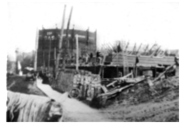
AFC 465-S3-I6 Distribution plant PUC front [under construction]. -- ca. 1905-1912. -- 1 b&w photograph (tiff, jpg)
