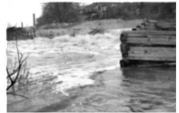
AFC 465-S13-I18 Floods on the Thames 2. -- ca. 1905-1912. -- 1 b&w photograph (tiff, jpg)
