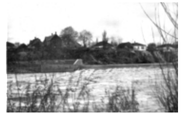
AFC 465-S13-I19 Floods on the Thames 3. -- ca. 1905-1912. -- 1 b&w photograph (tiff, jpg)
