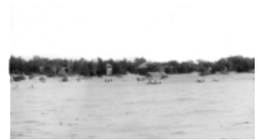
AFC 465-S10-I23 Grand Bend looking inshore. -- ca. 1905-1912. -- 1 b&w photograph (tiff, jpg)
